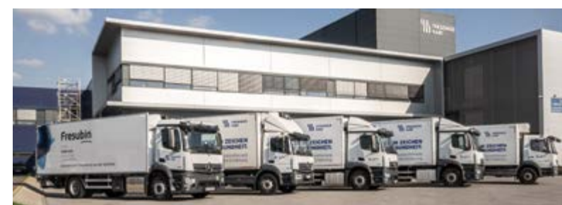
Das moderne Cargo-Center in Werndorf
